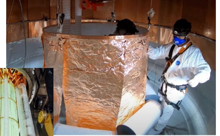
WaveLength-Shifting Reflector (WSLR) installed
