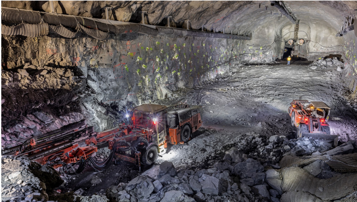
Drilling holes for blast charges for bench C (left) and removing muck (right) in North Detector Cavern (4850-33) west end
