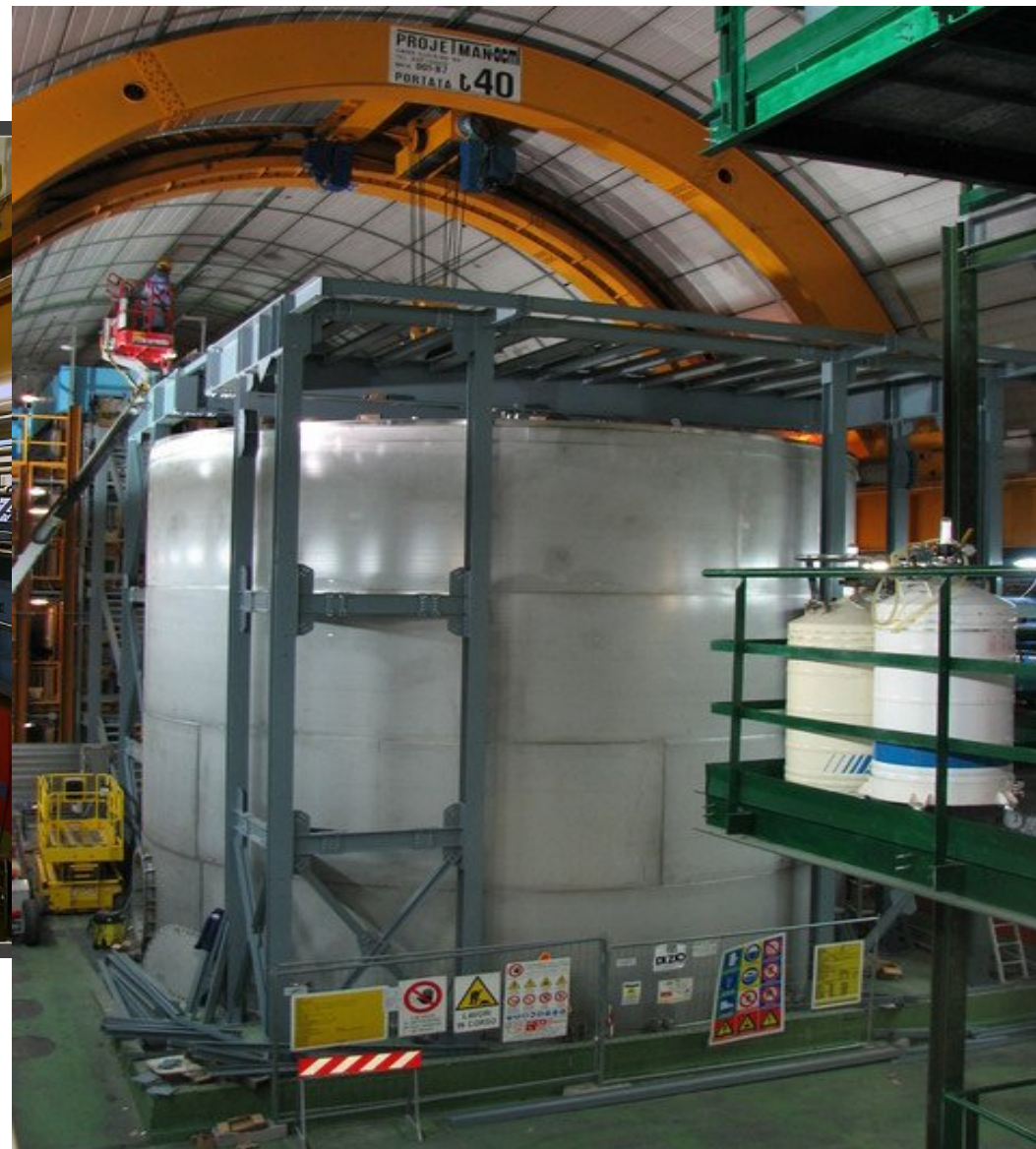
Watertank and Superstructure August 2008
