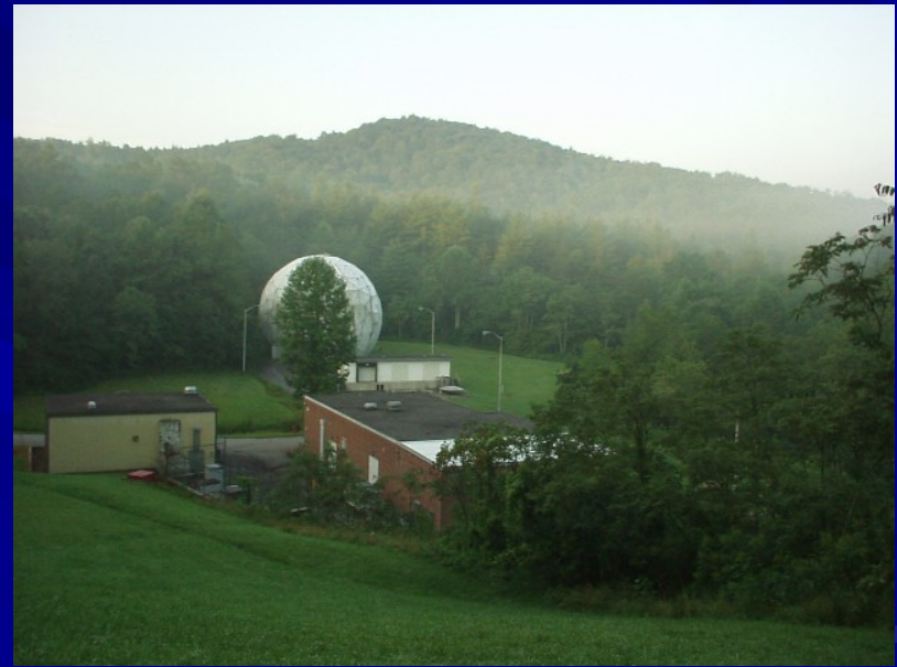
Array site near bottom of "bowl" formed by surrounding terrain
